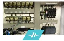
UL CSA listed electrical and instrumentation control panels, VFD and PLC driven panels, or Variable Speed Drive (VSD) panels to control and minimize transient pressures.
